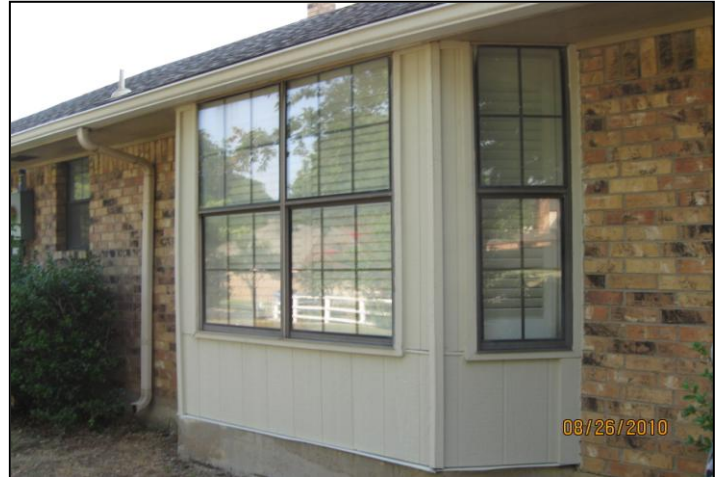
MHRP Siding Project
