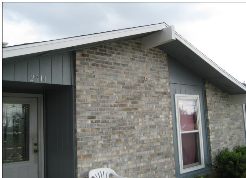
MHRP Painting and Siding Project
