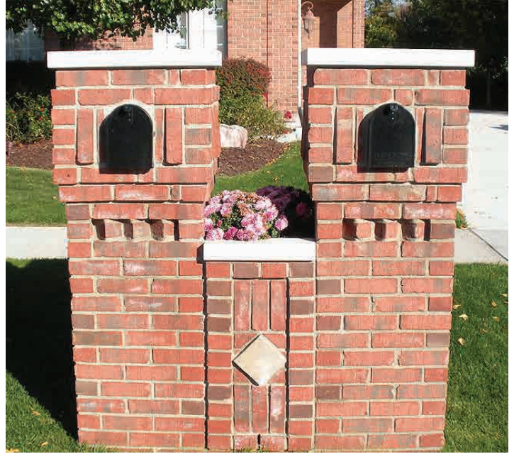
Paired masonry mailboxes help open up on-street parking.
