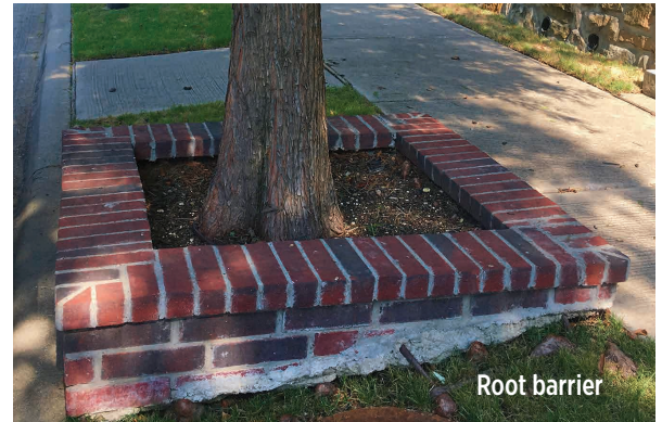
Root barrier required to be installed per the City of Carrollton's General Design Standards
