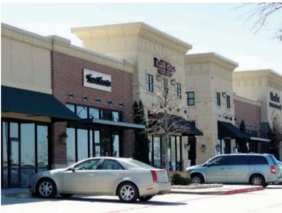
Repeat elements along each elevation.
