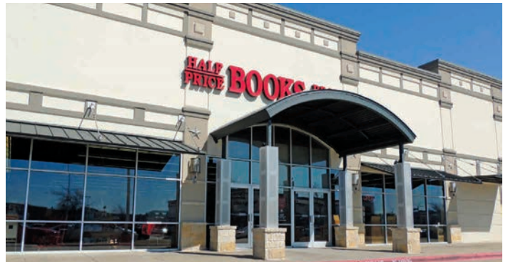
Storefront windows are more expansive.
