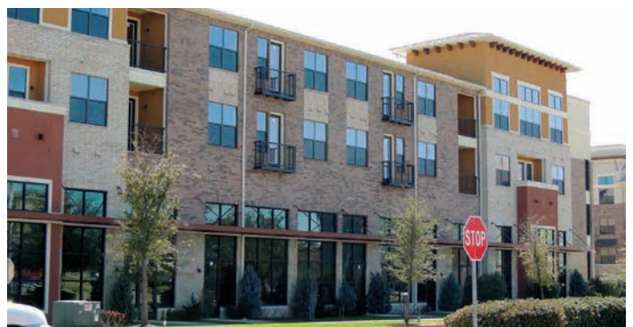
Window and doors narrate the uses inside.
