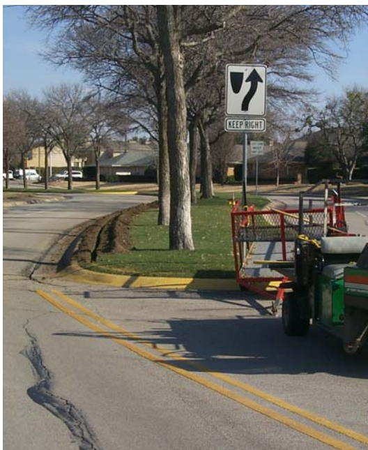
Improvements in progress
