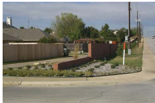
Completed project at Hebron & Arbor Creek
