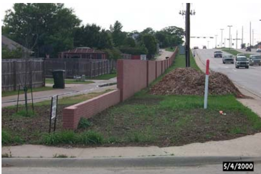
Project in progress at Hebron & Arbor Creek
