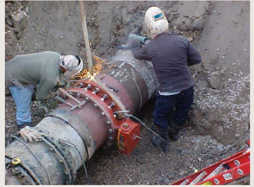
Major Water Distribution System Leaks Historical Data
