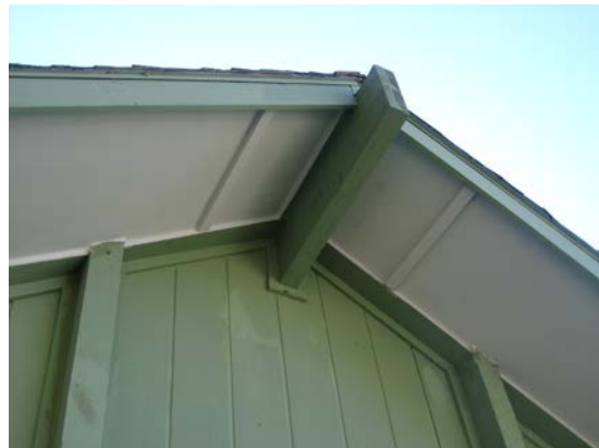
MHRP Siding and Paint Project
