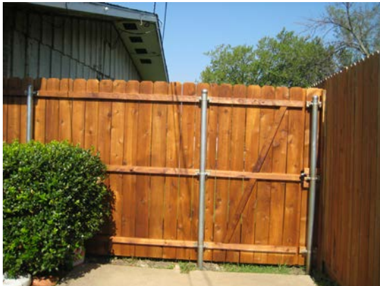
Public Service Fence Project
